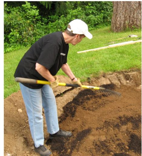
Schedule work when soils are dry to prevent compaction. Photo: Erica Guttman
