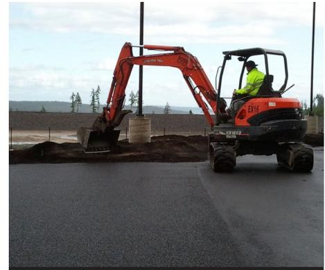
Newly installed pervious pavement must be protected prior to constructing an adjacent rain garden to prevent soils from clogging the pavement. Photo: Erica Guttman
