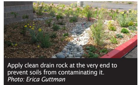
Apply clean drain rock at the very end to prevent soils from contaminating it. Photo: Erica Guttman
