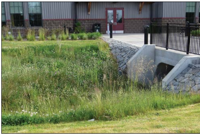
Figure 2. A water catchment swale (left) at the Oldfield Animal Teaching Facility on the campus of Oregon State University has grasses and clover, and mimics a natural site by slowing and filtering water flowing through the landscape. The rest of the landscaping (right) is conventional, however, and provides few additional ecological services. An ecological design of native plants in both the swale and the rest of the site could have reduced mowing and irrigation, provided wildlife habitat, and created a more interesting and aesthetically pleasing landscape.
