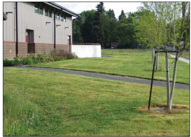
Figure 2. A water catchment swale (left) at the Oldfield Animal Teaching Facility on the campus of Oregon State University has grasses and clover, and mimics a natural site by slowing and filtering water flowing through the landscape. The rest of the landscaping (right) is conventional, however, and provides few additional ecological services. An ecological design of native plants in both the swale and the rest of the site could have reduced mowing and irrigation, provided wildlife habitat, and created a more interesting and aesthetically pleasing landscape.
