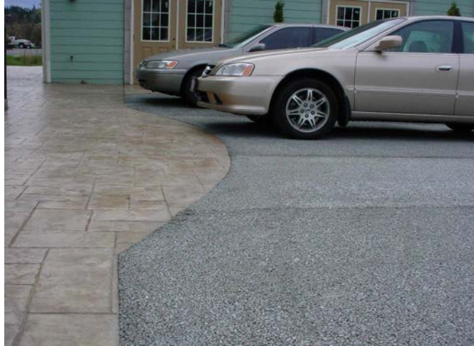
Clear example of edging between traditional impervious pavement and a permeable pavement parking lot
