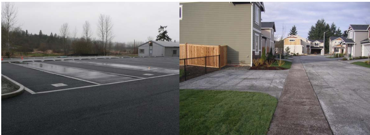
Examples of wearing courses – porous asphalt (left) and pervious concrete (right)
