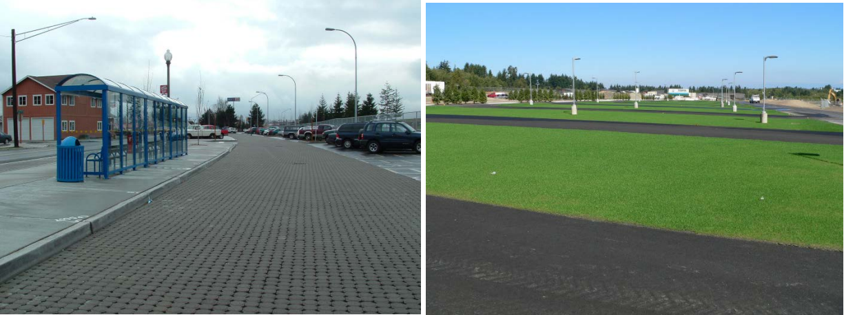
Examples of wearing courses – pavers (left) and grid with grass (right)
